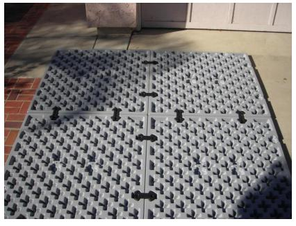
Drive two screws into each of eight EZ Pad connectors.
